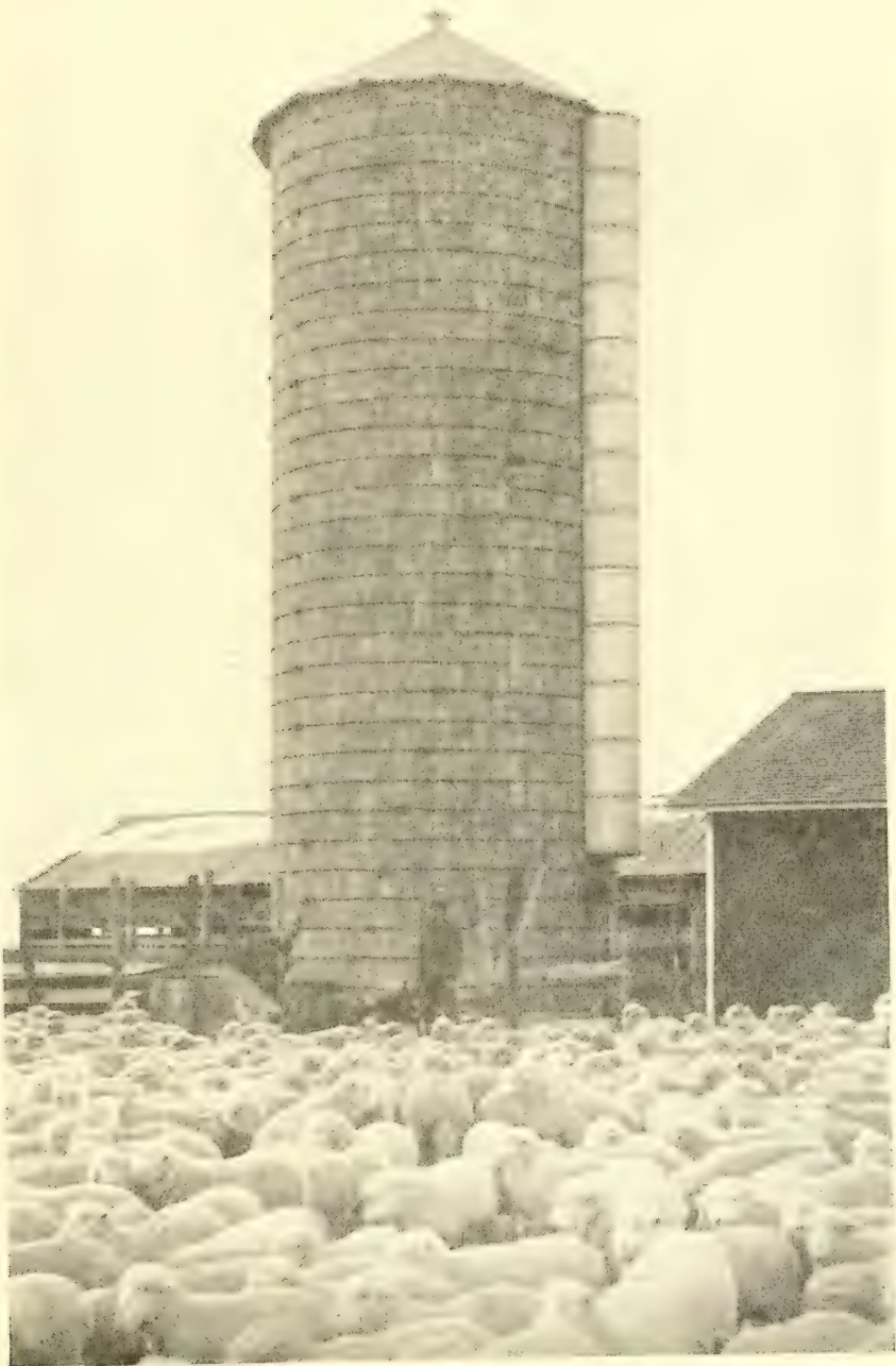
Playford Cement Stave Silo. (131)
